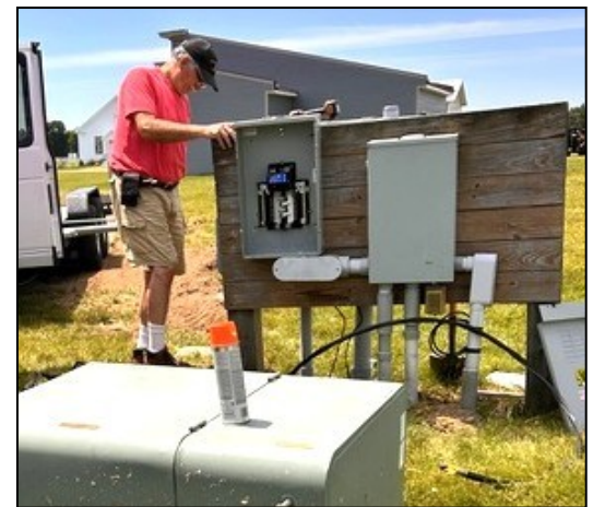
Jay Foster at work on the electrical system.
