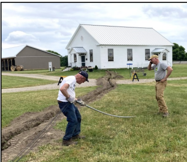
Lee Gooden (l) and Robert Crump pulling cable into conduit.
