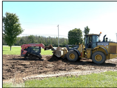
Construction of tracks at the Museum for Locomotive 210 began with grading (left) and setting the sub-ballast (right) consisting of 12 inches of compacted no. 3 stone. Enough has been completed to accommodate laying of 100 feet of ties and rails in the near future, more than enough for delivery of the 210.
